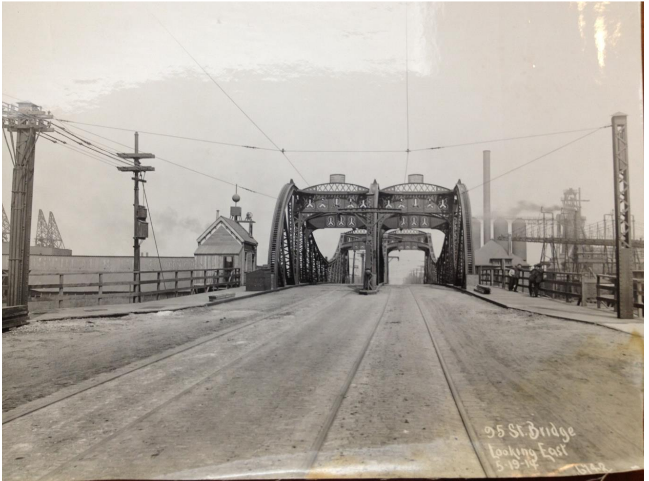
Old bascule bridge at 95 th Street, 1914. Chicago Bridges Collection, Chicago History Museum.
