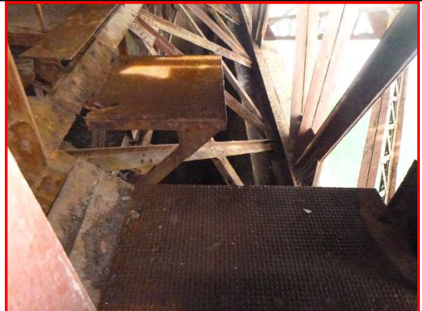
76. West pit catwalk steel plating, looking north.
