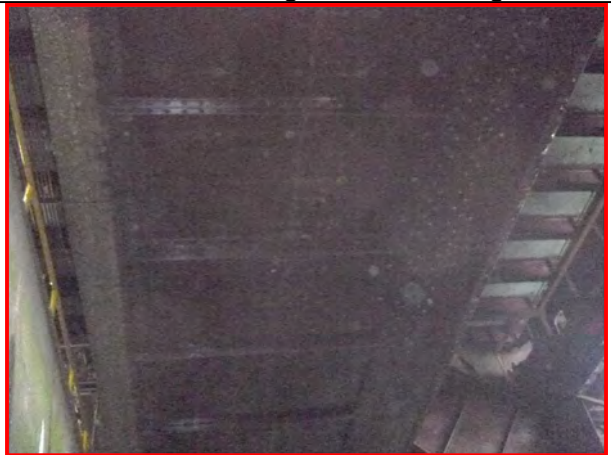
71. Bottom of west counterweight box, looking north.
