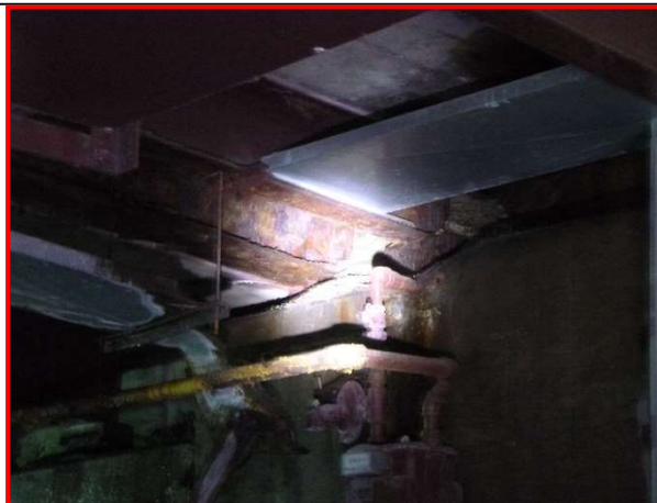
35. East Abutment bearings, looking east.
