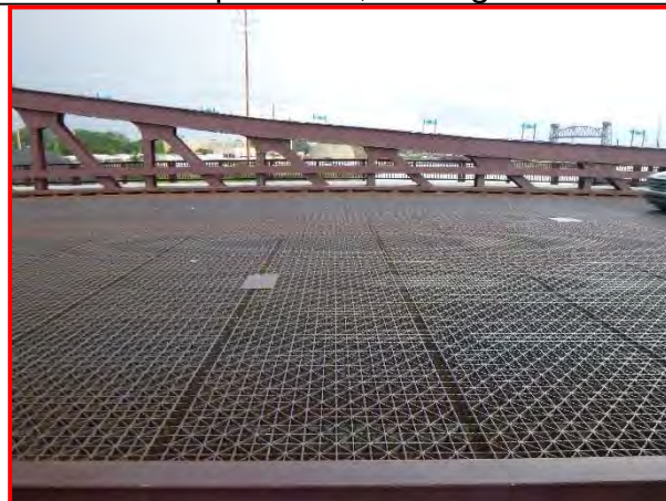
3. Steel plate repairs along the open steel grating, looking northeast.
