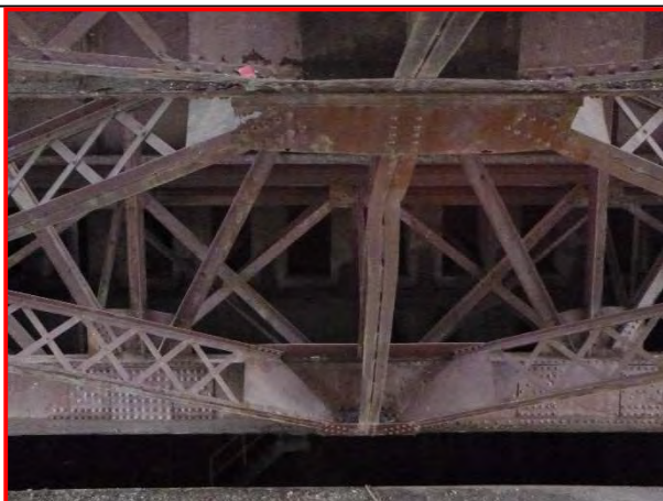
61. Panel 1 lateral bracing, looking east.
