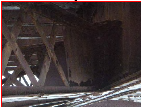
60. Panel 13 Lateral bracing stiffener plate, looking west.
