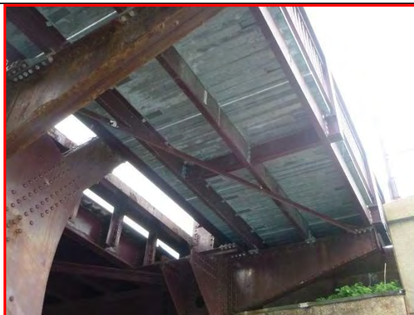
50. Span 2 south sidewalk stringer, looking northeast.
