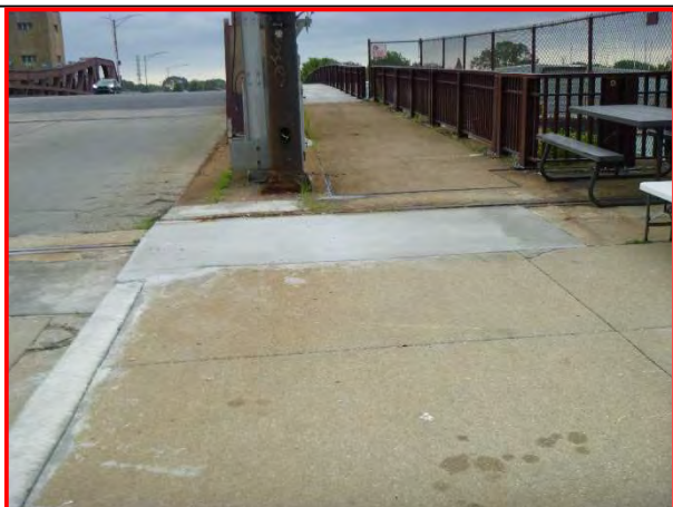
18. Southwest approach sidewalk, looking east.
