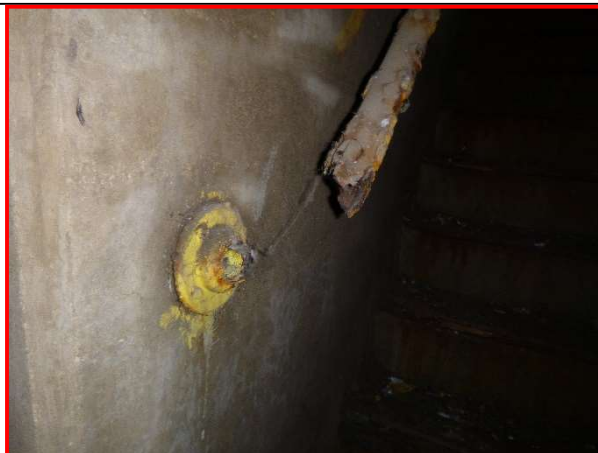
73. Railing in west bridge house, looking southeast.
