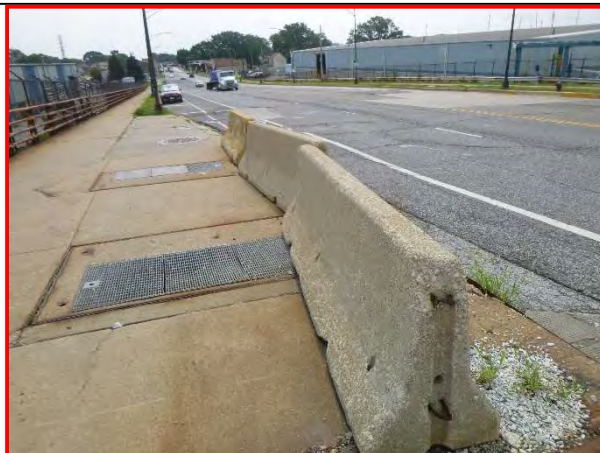
27. Temporary concrete barriers along northeast sidewalk, looking east.
