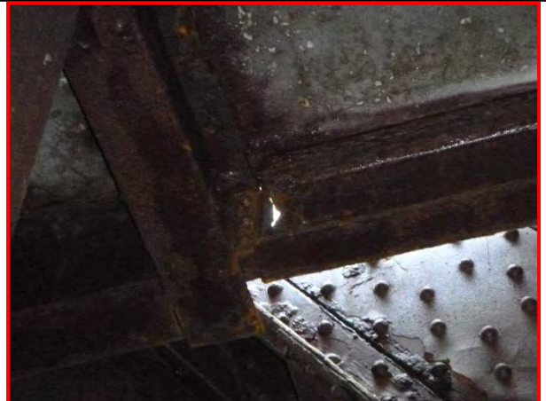
41. Span 4 south sidewalk stringer, looking north.
