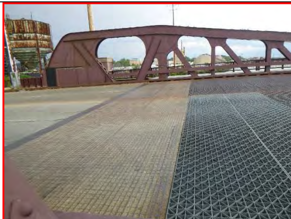
4. Span 3 interface of concrete filled and open steel grating, looking north.
