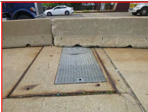
19. Typical fixed span sidewalk, looking east.
