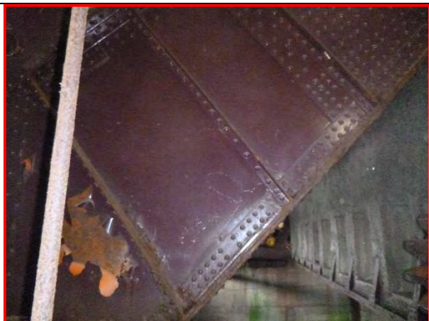
52. Southeast trunnion girder, looking north.
