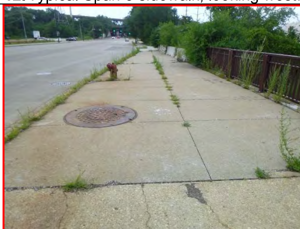
14. Northwest approach sidewalk, looking west.
