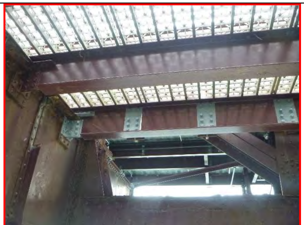
44. Panel 7, Stringer 1, looking south.
