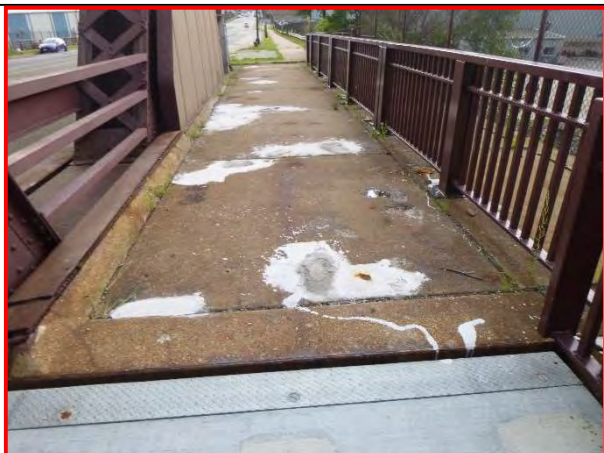
16. Spans 1 and 2 sidewalk, looking east.
