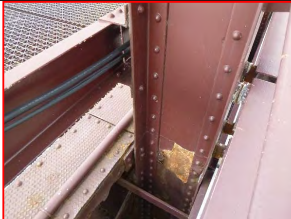
67. Bottom chord member at northwest support, looking west.
