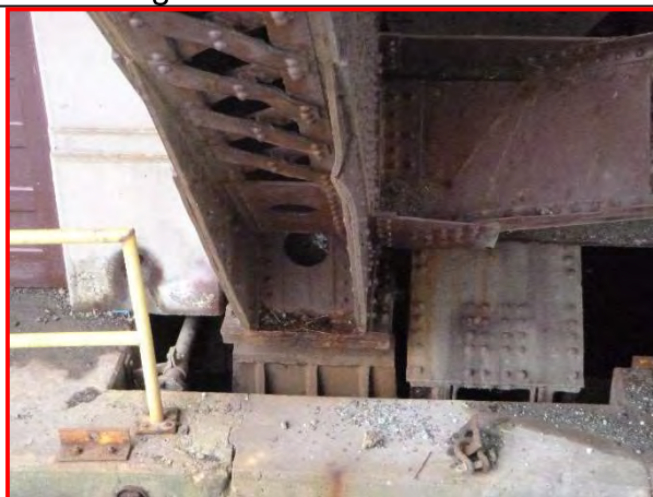
66. Bottom chord member at northeast support, looking east.
