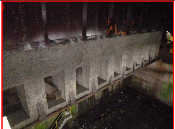
70. East counterweight box, looking east.
