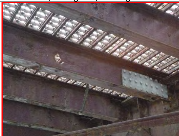
48. Panel 12, Stringer 6, looking southwest.
