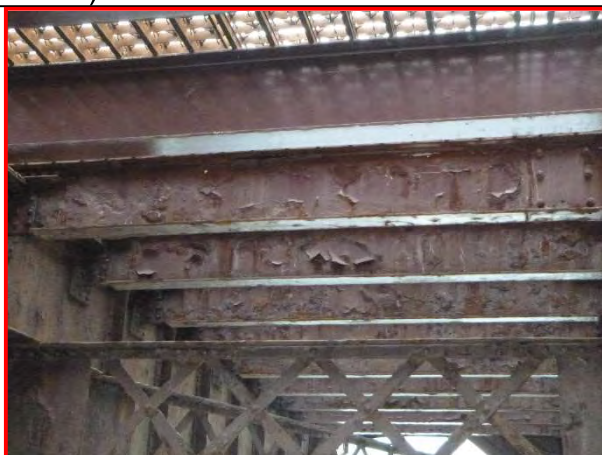
43. Panel 8 stringers, looking north.
