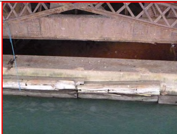
82. West fender, looking west.
