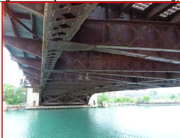
33. Overall underside of the movable superstructure, looking northwest.
