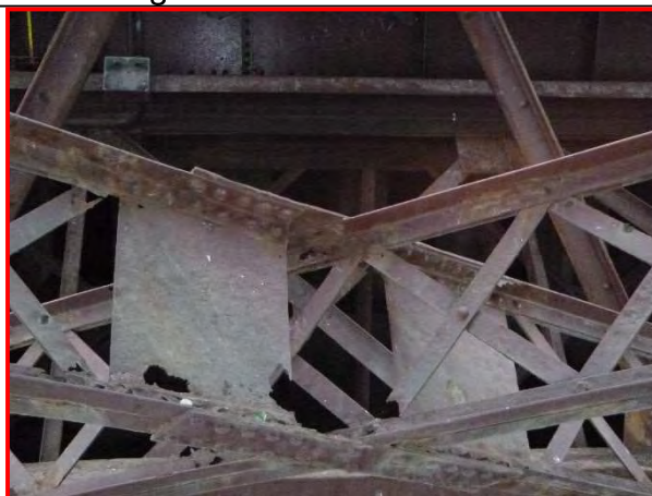
62. Panel 1 lateral bracing, looking east.
