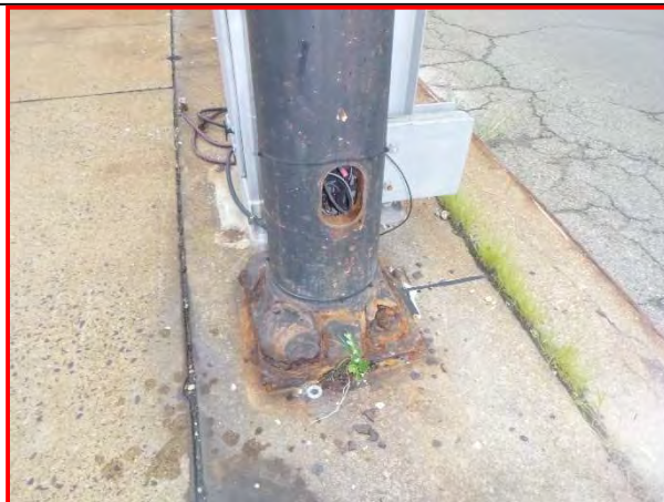
20. Typical light standard base, looking east.
