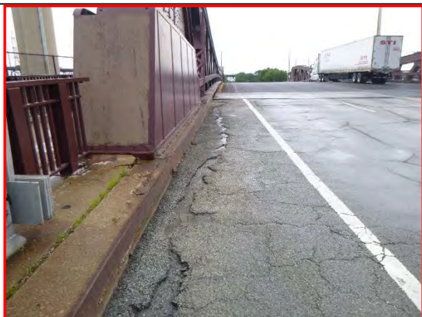
6. Span 2, south curb, looking west.
