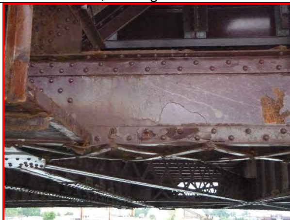
64. Panel 7, south bottom chord member, looking north.
