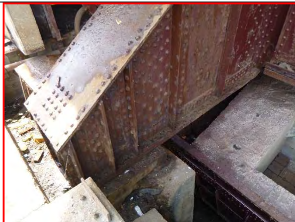
39. Southwest longitudinal girder bearing, looking south.
