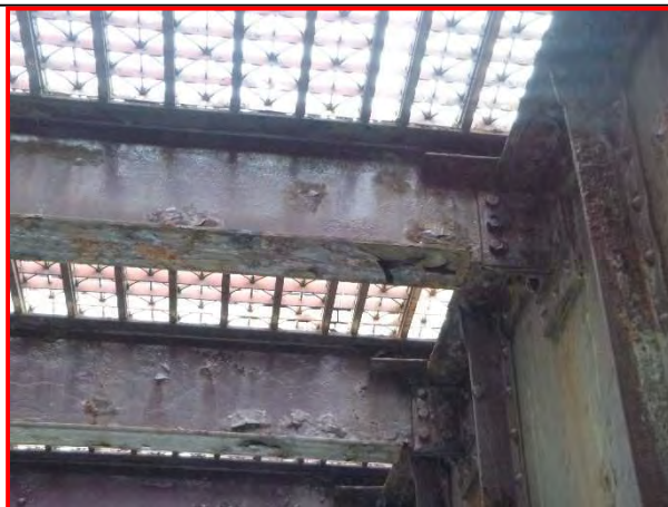
84. Typical moveable span paint system, looking north.
