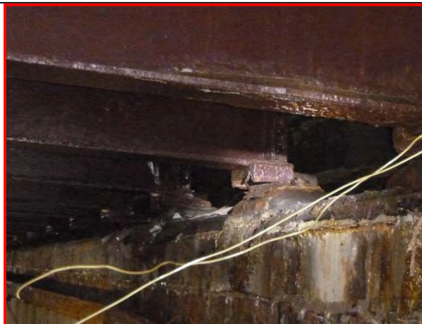
34. West Abutment bearings, looking southwest.
