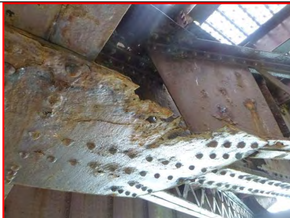
63. Floorbeam 2W Lateral bracing connection, looking west.
