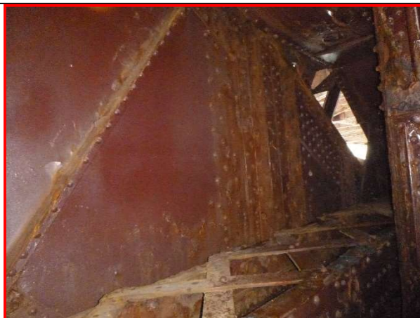
53. Vertical stiffeners of the southeast trunnion girder, looking east.
