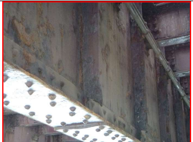
56. Typical moveable span floorbeam, looking southeast.
