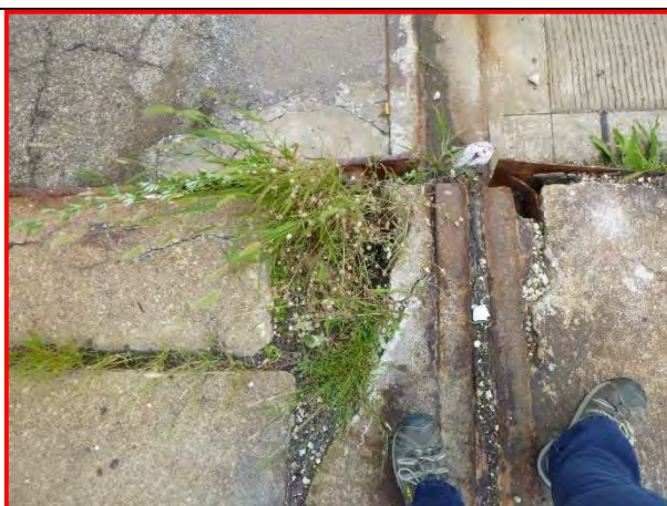
13. North sidewalk at West Expansion Joint, looking down/south.
