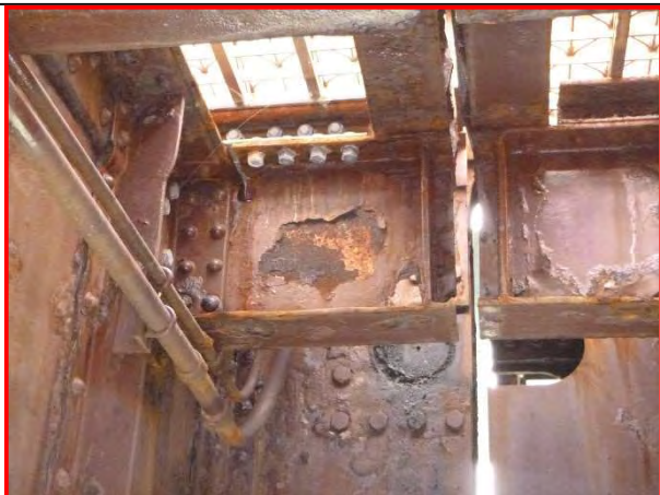
45. Panel 8, Stringer 1, looking south.
