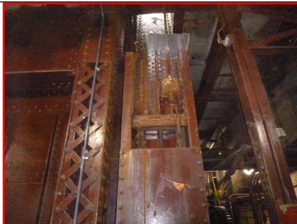
38. Northeast secondary live load bearing, looking west.
