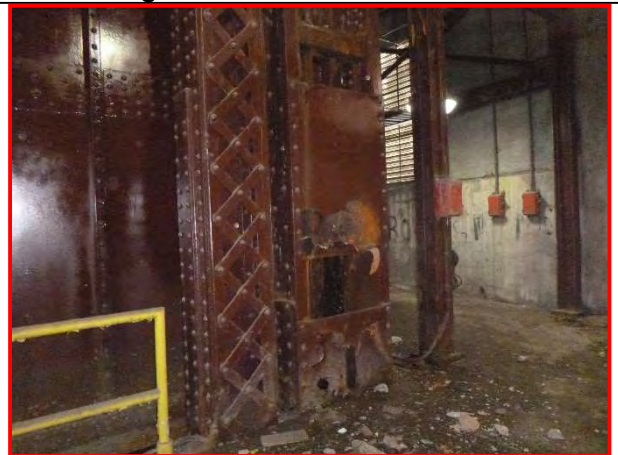
86. Typical substructure paint system, looking southeast.
