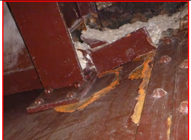
55. South end of floorbeam 21W, looking northeast.
