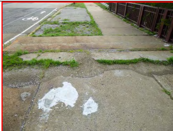
15. South sidewalk at east expansion joint, looking east.
