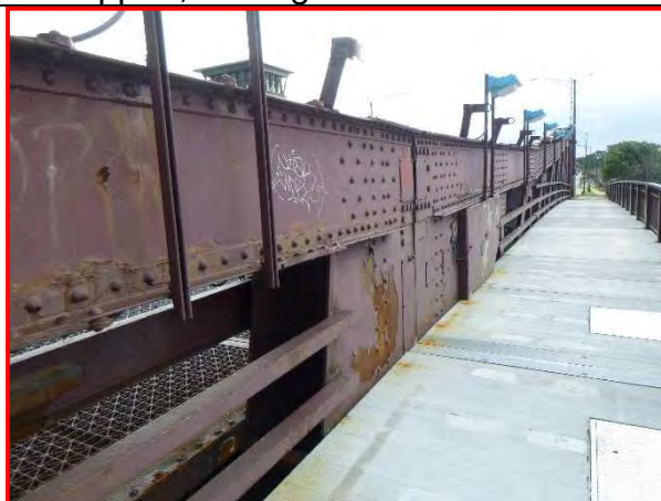
68. Top chord of south truss, looking northeast.
