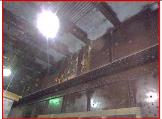
85. Typical fixed span paint system, looking southeast.
