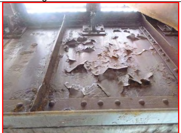
58. West end of FB 0W, looking east.
