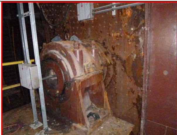
36. Southeast trunnion bearing, looking northwest.
