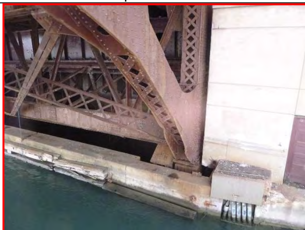
65. Bottom chord member at northwest support, looking west.
