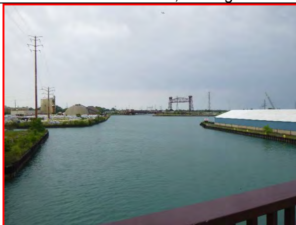
88. Upstream channel, looking north.
