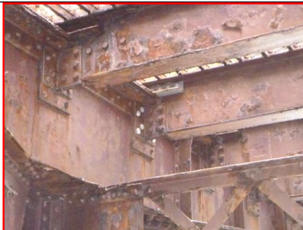
46. Panel 9, Stringer 9, looking southeast.
