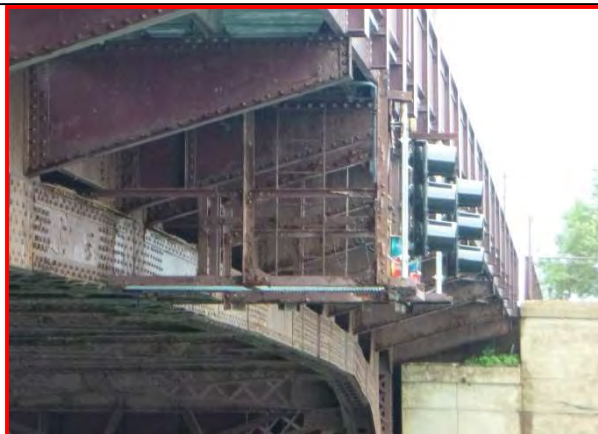
75. Catwalk on south truss, looking east.
