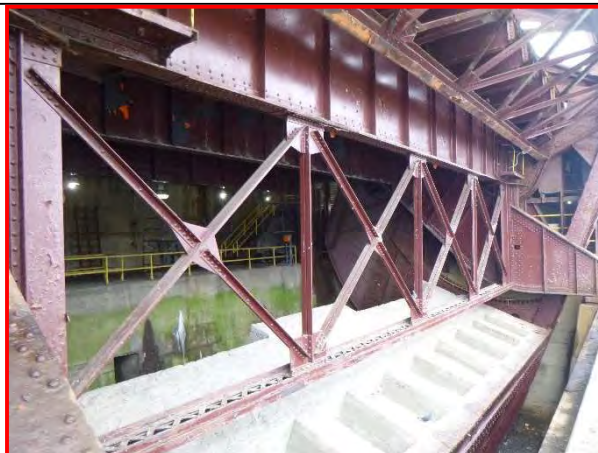
51. Southeast trunnion girder, looking south.
