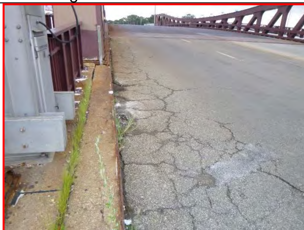
7. Span 4, north curb, looking east.
