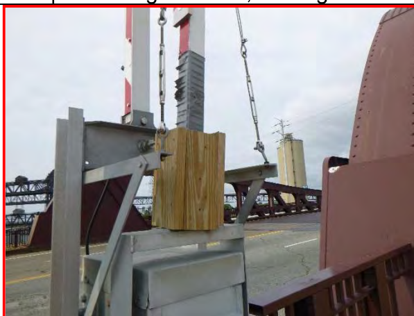
32. Span 1 northeast traffic barrier, looking southwest.
