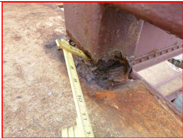
5. Northwest rail post, looking south.
