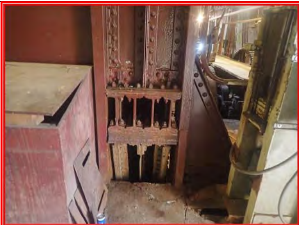
78. Northwest anchor column, looking south.
