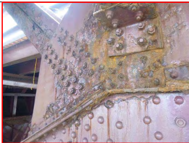
54. Gusset plate 8, southeast truss, looking west.
