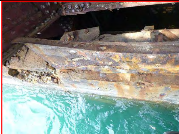
73. Steel guard rail on the north river pier, looking north.
