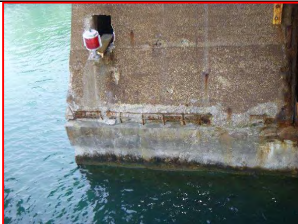
65. South bridge house at the water line, looking south.
