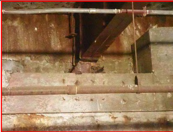
29. Stringer 9 bearing at South Abutment, looking south.
