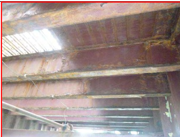
83. Superstructure paint, looking east.
