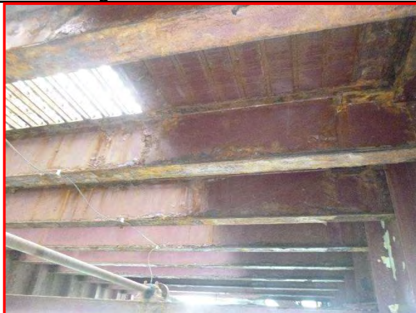
33. Typical movable span roadway stringer, looking east.
