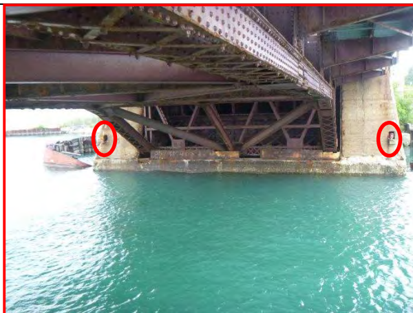
82. Navigation lights on the south river pier, looking south.
