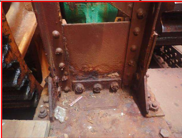
84. Substructure paint system, looking down.
