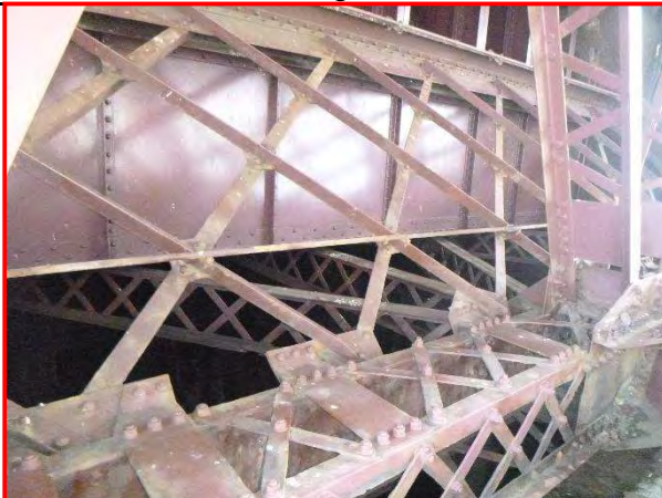
45. Southwest lattice truss, looking south.
