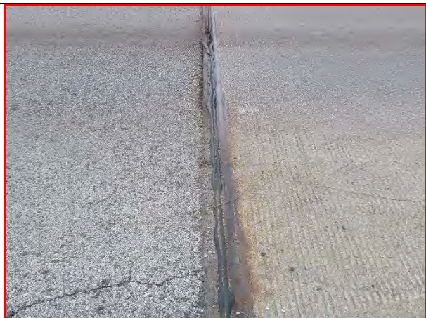
22. North approach expansion joint, looking northeast.
