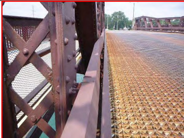
7. West brush rail, Span 3, looking north.
