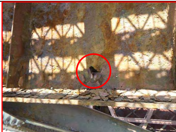
43. Floorbeam 8-8N, looking northwest.
