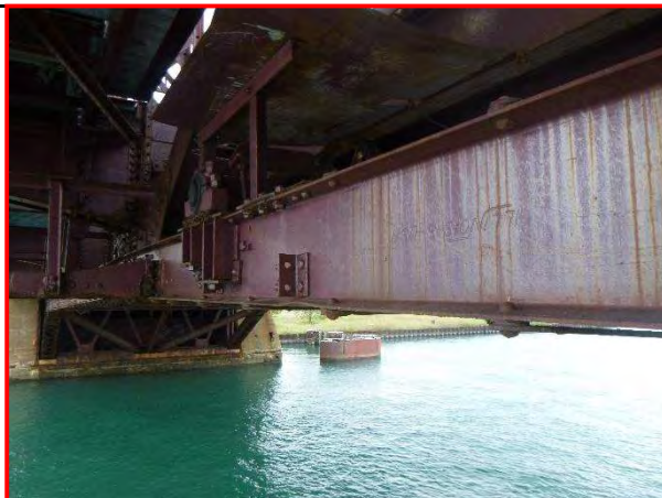
51. Northeast truss, member 0-2, looking southwest
