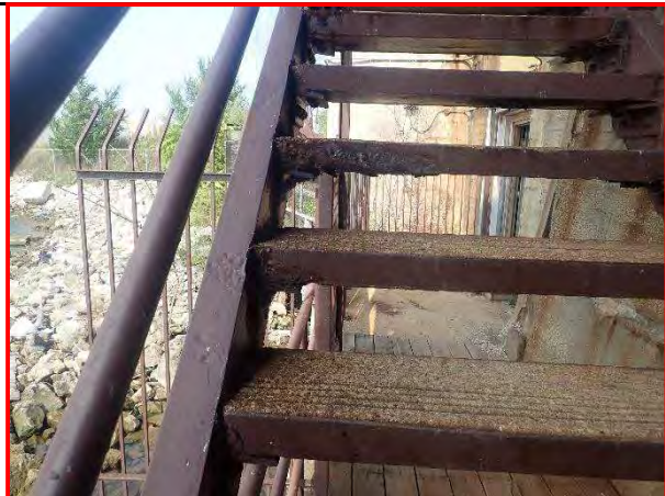
66. Northwest stairwell, looking north
