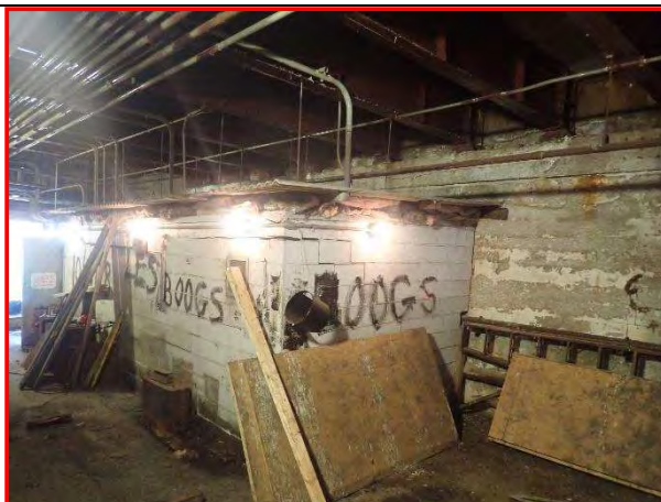
70. South Abutment, Looking southeast.
