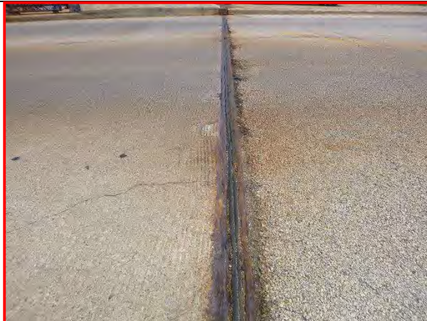
14. Typical south expansion joint, looking east.
