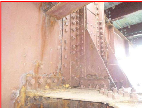
44. Typical condition of anchor column floorbeam, looking northwest.
