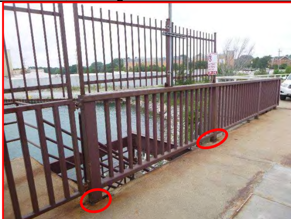
4. Northwest railing, looking west.
