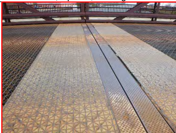
9. Median, Span 3, looking east.
