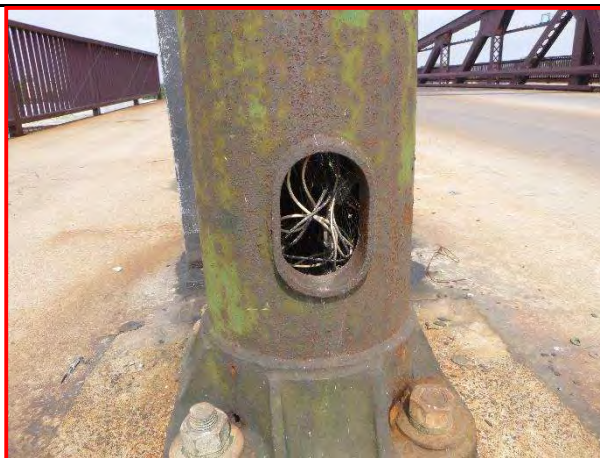
11. Typical light standard base, southwest corner, looking north.
