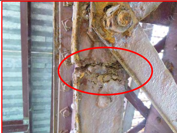
56. Bottom chord 2-4, southeast truss, looking up.
