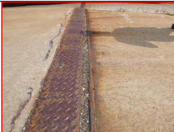
15. Southwest sidewalk expansion joint, looking east.
