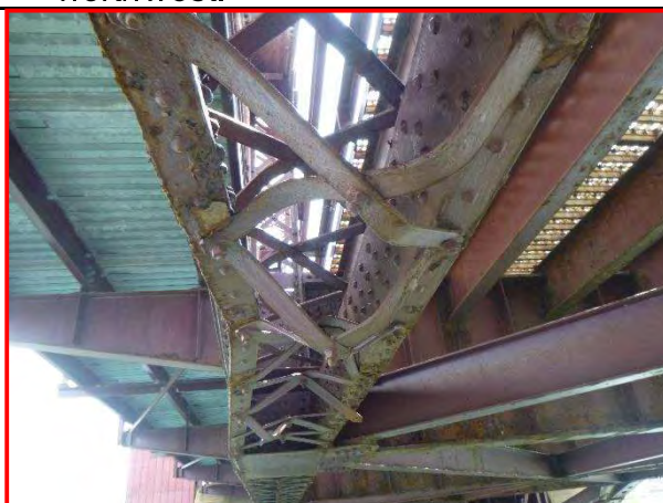
49. Bottom chord, member 2-4SE, looking south.
