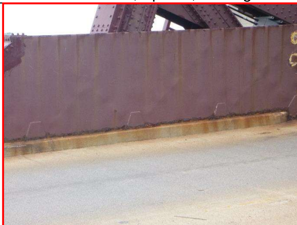
8. East curb, Span 1, looking east.
