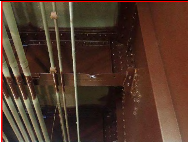
36. Span 5, Stringer 5 at anchor column girder, looking west.
