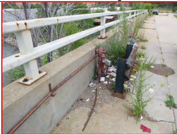
25. Gas Utility, northwest approach sidewalk, looking northwest.
