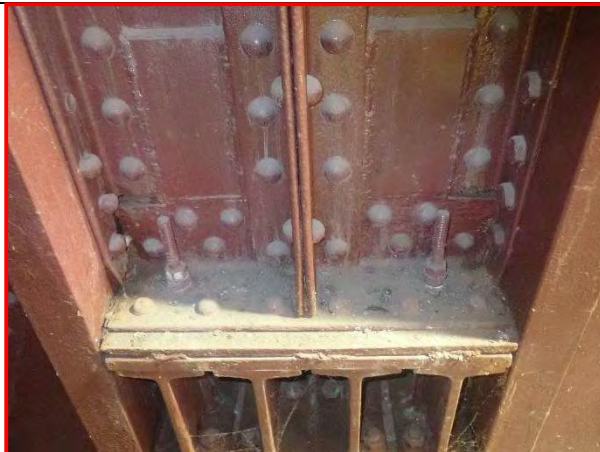
79. Southwest anchor column, looking north.
