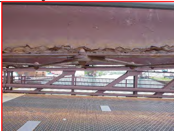
59. Typical top chord member, west truss, looking east.
