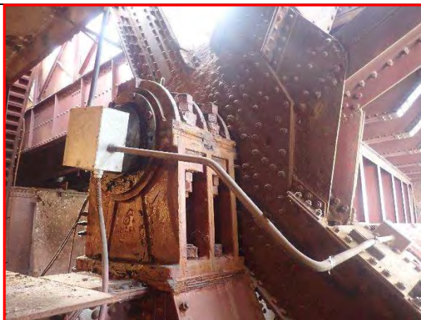
31. Typical trunnion bearing, looking southwest.
