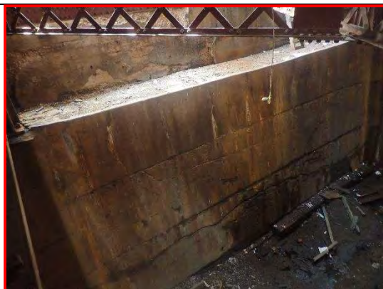
74. View of north face of north river pier, looking south.
