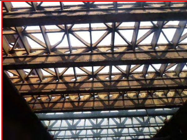
18. Span 3 underside, looking north.
