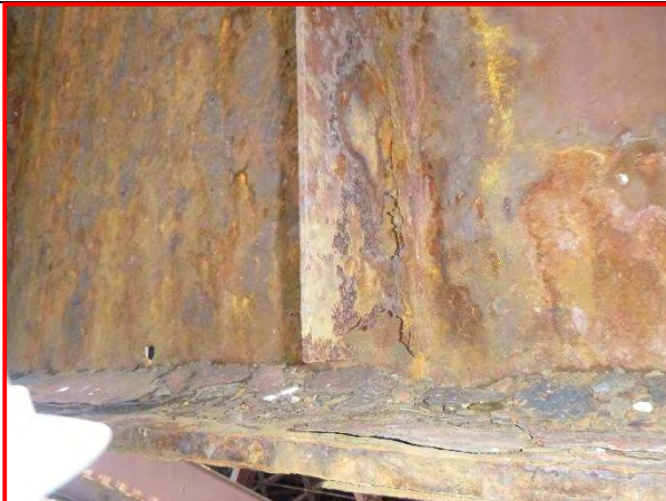
42. Floorbeam 8-8S stiffener, looking south.
