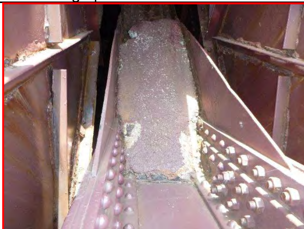
57. Truss member B-12, southeast truss, looking south.
