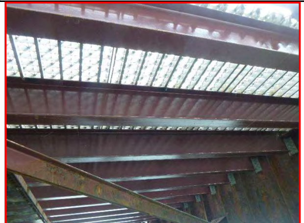
37. Panel 1, between floorbeam 8 and 10, looking northeast.
