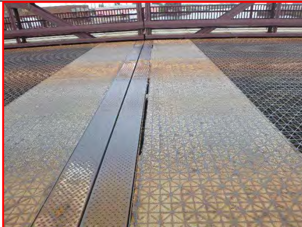
3. Concrete filled section along center break, looking east.
