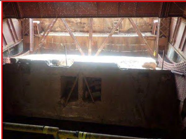
64. Top of north counterweight, looking south.
