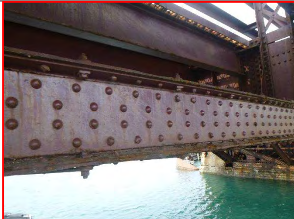
48. Bottom chord, northeast truss, looking northwest.
