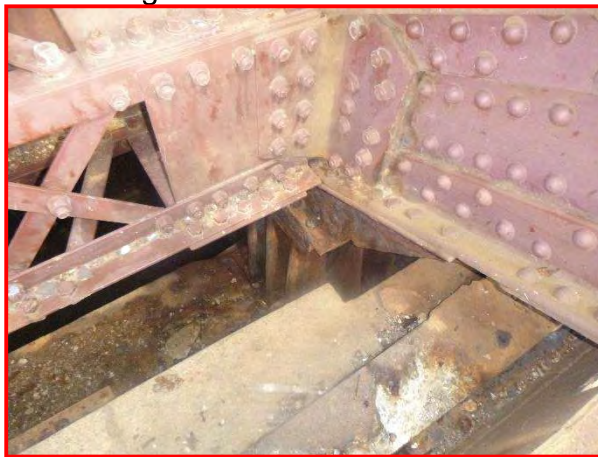
30. Northeast live load bearing, looking north.
