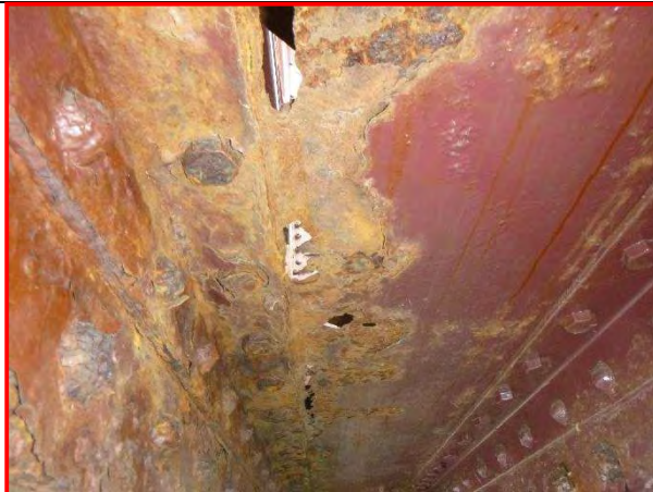
52. Batten plate of bottom chord 4-6, northwest truss, looking north.
