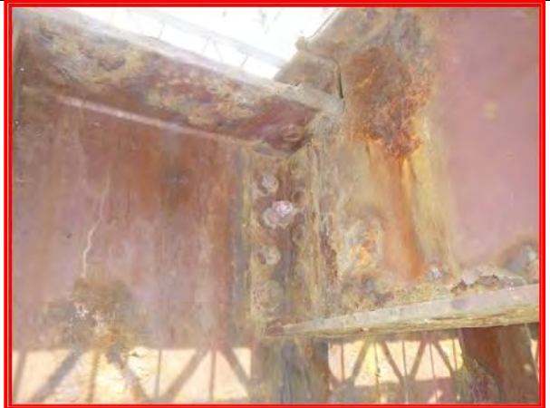
35. Typical stinger to floorbeam connection, looking north.
