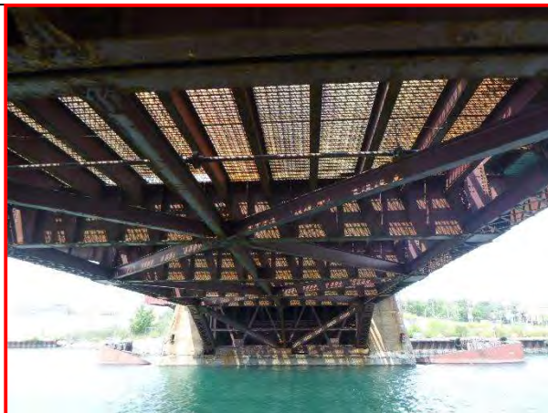
28. Overall underside, looking north.
