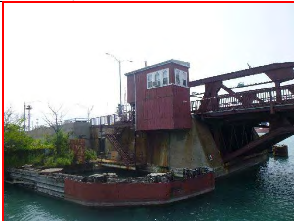
67. Overall Northwest bridge house, looking northeast.
