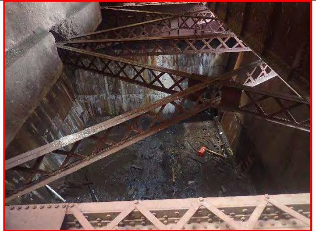
46. Typical lateral bracing over counterweight pits, looking west.
