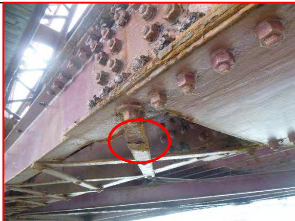
50. Typical lacing bars, looking southwest.
