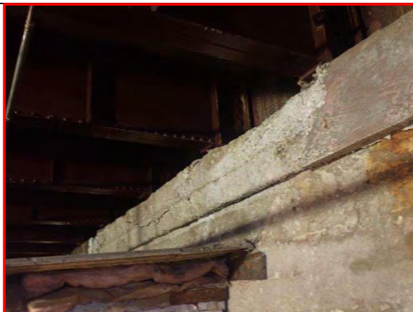
72. South Abutment bearing seats, looking southeast.
