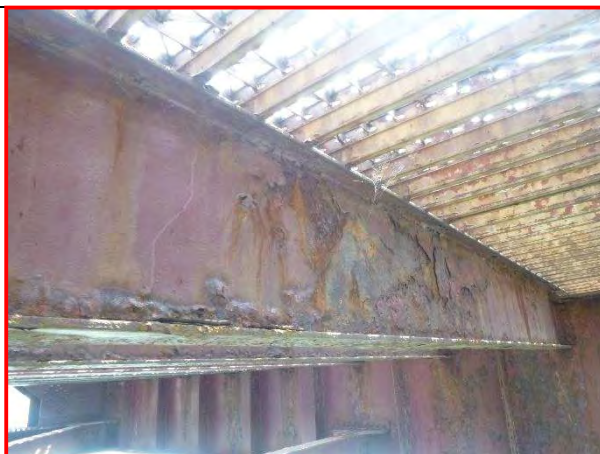
34. Stinger 8, north leaf, between floorbeams 4 and 6, looking south.
