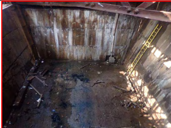
80. North counterweight pit walls, looking east.
