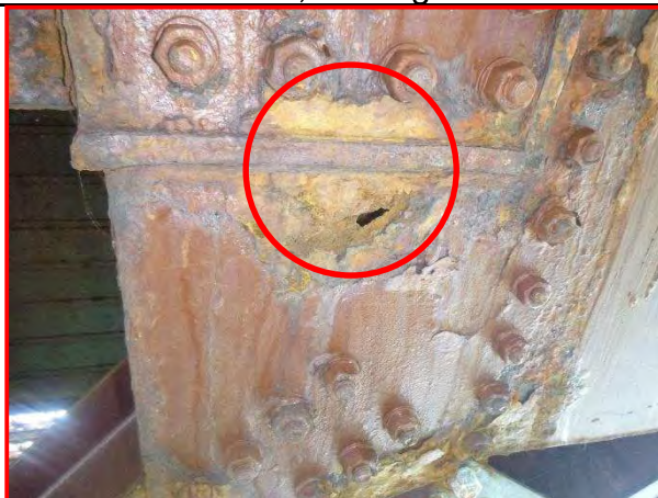
53. Bottom chord 0-2 and lateral bracing connection, southwest truss, looking west.
