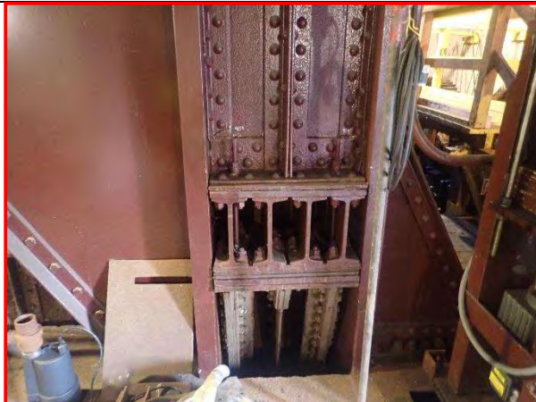
76. Southeast anchor column, looking north.
