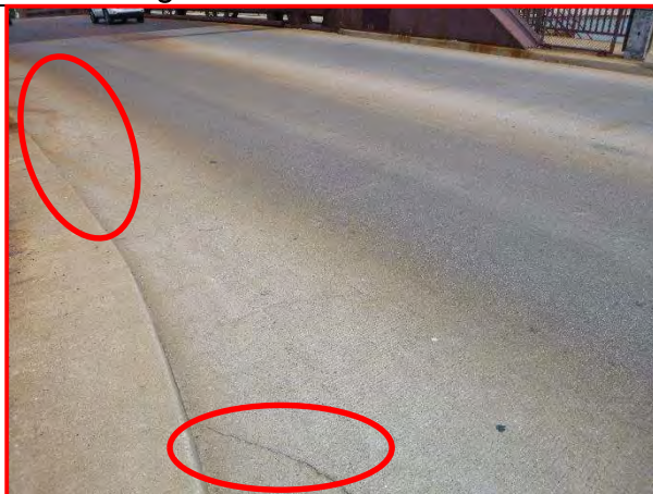
2. Typical bare concrete deck, fixed span, looking southeast.
