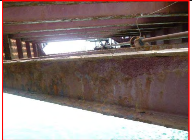
47. Lateral bracing, north leaf, looking east.
