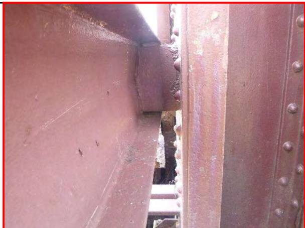
58. Truss and steel angle connection, looking southeast.
