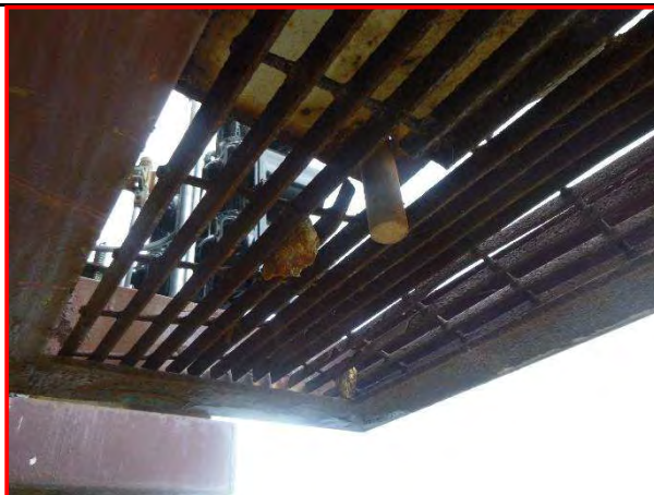
69. Southeast catwalk, looking north.
