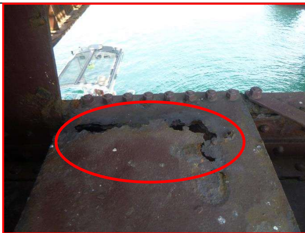
55. Batten plate, southwest truss, looking southeast.
