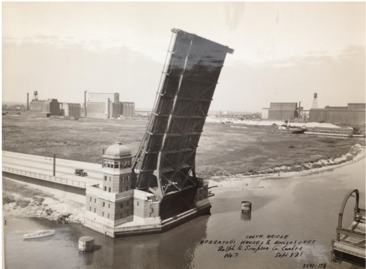
106 th Street Bridge, September 7, 1931. Department of Public Works Photo Collection, 1860-1948, Chicago History Museum.
