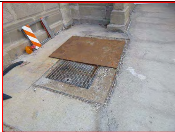
11. Steel plate in the northwest sidewalk, looking west
