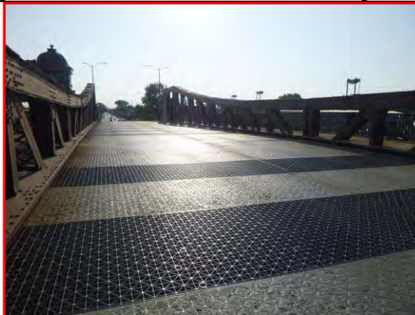
1. Overall top of deck, looking southeast
