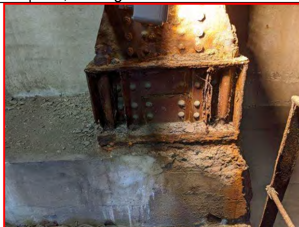
67. Northwest trunnion girder column base, looking north
