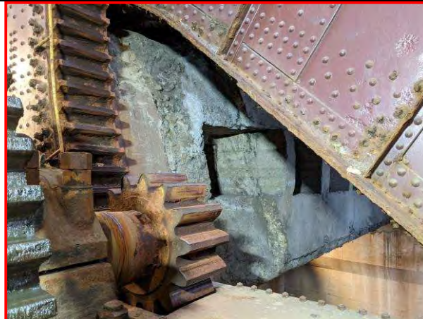
51. West counterweight box concrete, looking northwest
