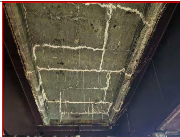
15. Span 1 soffit, looking east
