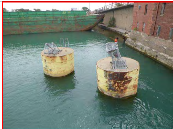
63. Northeast dolphin, looking east
