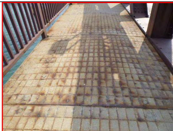
8. South sidewalk, looking west
