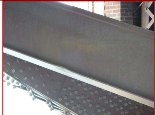
36. Lateral bracing between Floorbeam 14W and 16W
