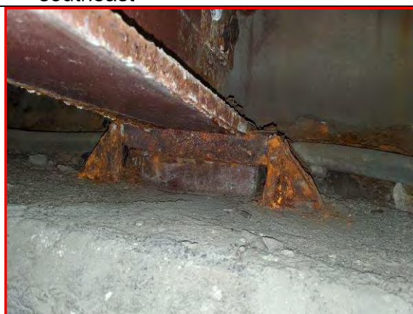
26. East Abutment bearing, looking northeast
