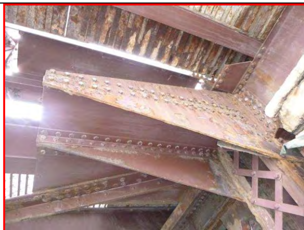
46. Gusset plate 16A NW, looking southwest
