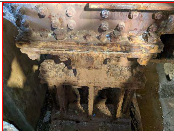
25. NW live load bearing, looking southeast
