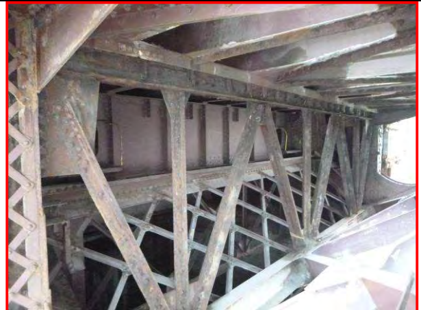
34. Floorbeam 16-16E, looking southeast
