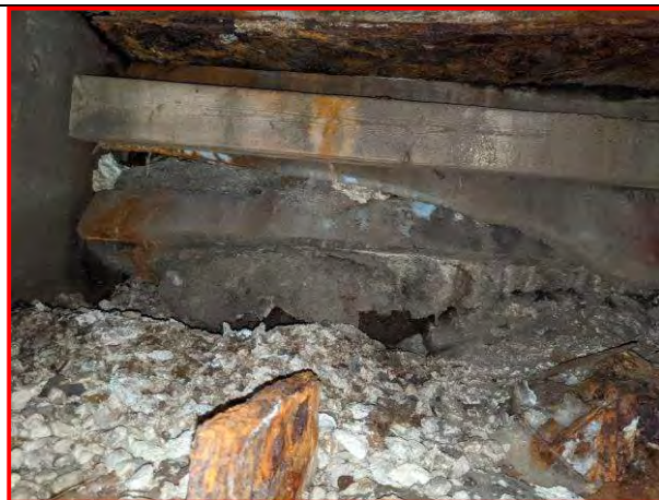
56. West Abutment backwall, looking west
