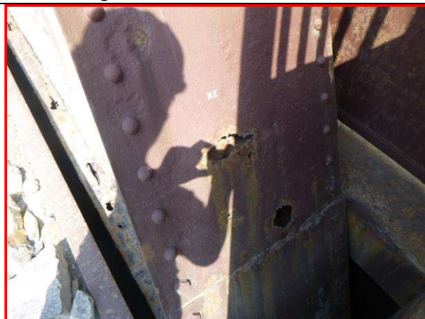
49. Northeast curved truss member, looking west
