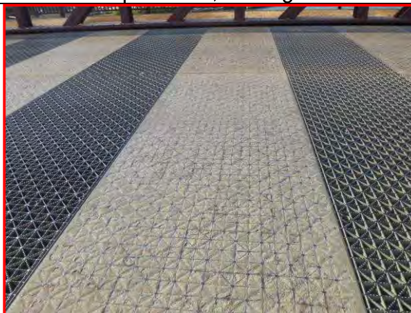
2. Typical movable wearing surface, looking south
