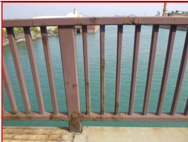
5. North steel rail, looking north
