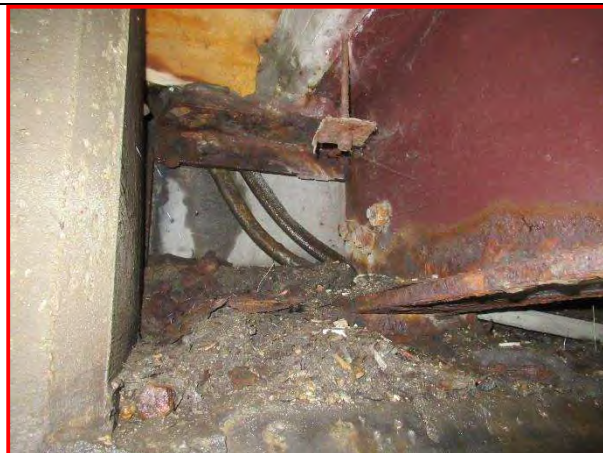
28. Span 5 stringer ends, looking west
