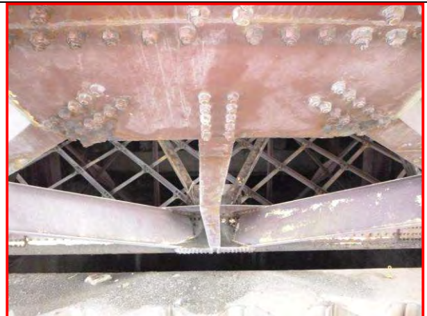
35. Lateral bracing between Floorbeam 12E and 14E, looking east
