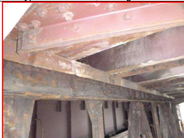
33. Floorbeam 14-14E, looking east
