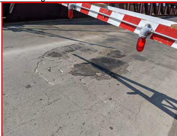
4. East fixed span wearing surface, looking southwest
