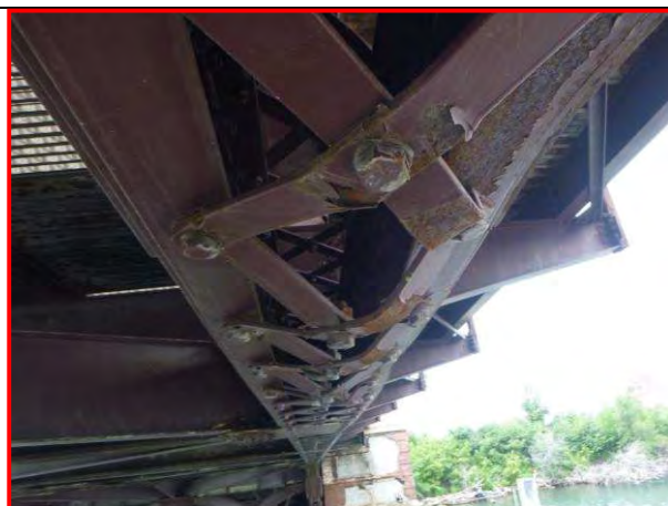
39. Bottom chord 2-4NW, looking south
