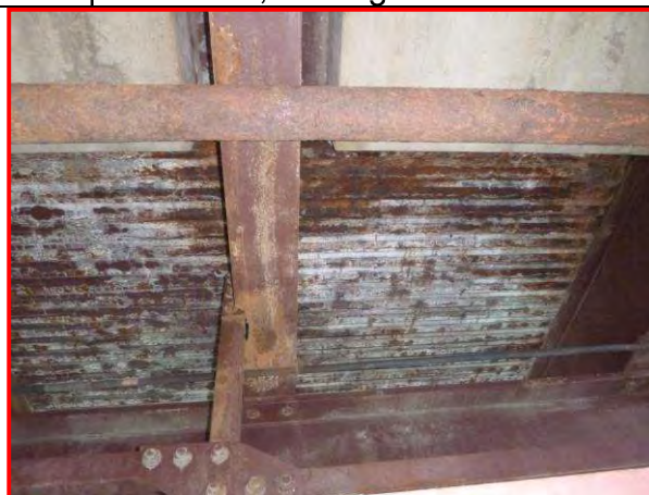
16. Span 3 soffit, looking east
