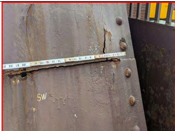
48. Southwest curved truss member, looking east
