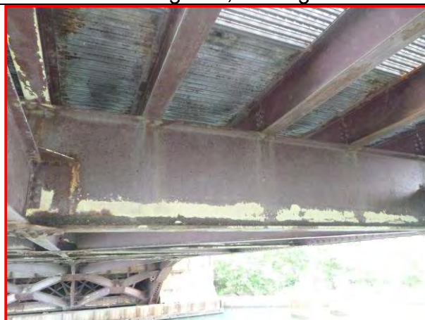
32. Typical floorbeam, looking southeast
