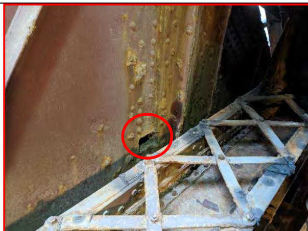
31. NE trunnion girder, looking southwest
