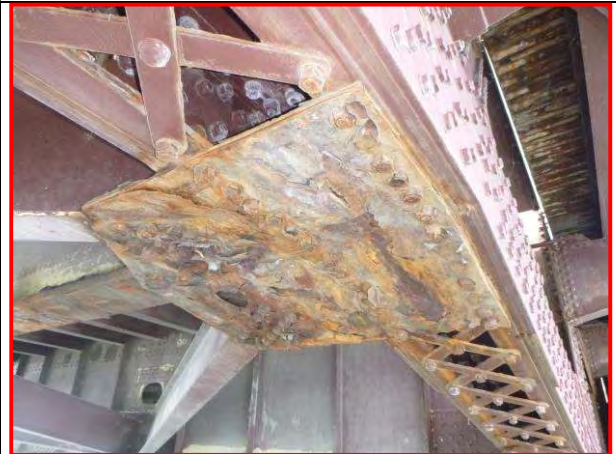
37. Lateral brace connection plate, looking southwest
