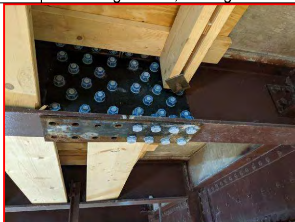
29. North sidewalk stringer in Span 4, looking south
