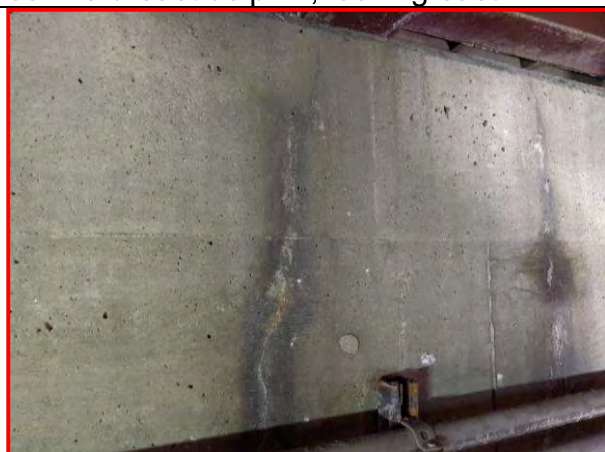
64. West Abutment wall, looking northwest
