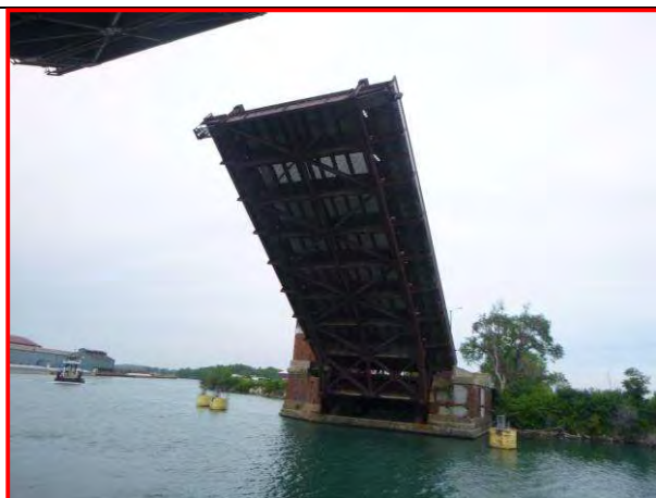
23. Overall underside of the movable superstructure framing, looking southwest
