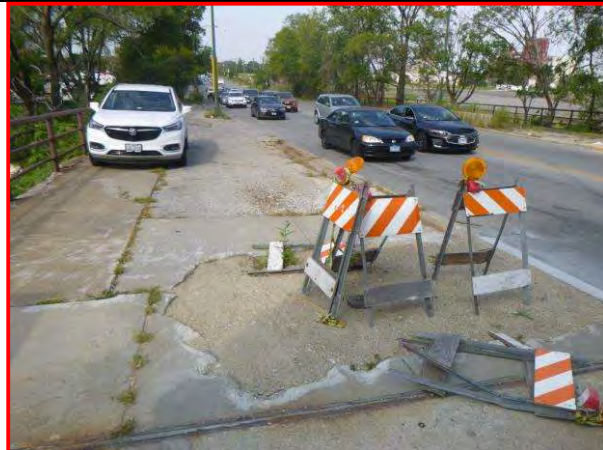
18. Edge of the southwest approach sidewalk, looking east
