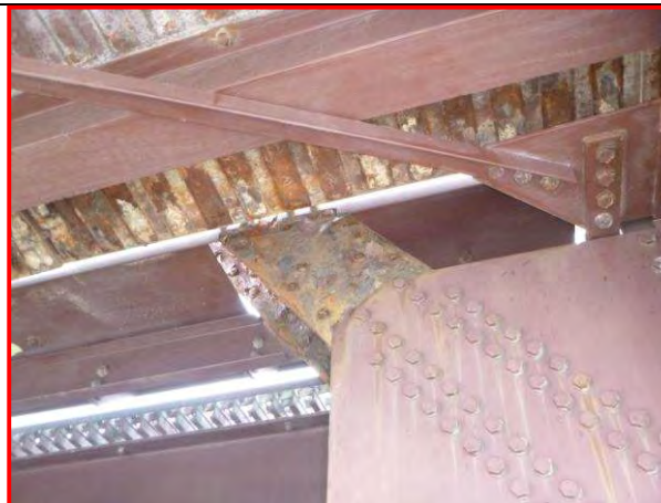
66. Southwest truss diagonal and gusset plate, looking north
