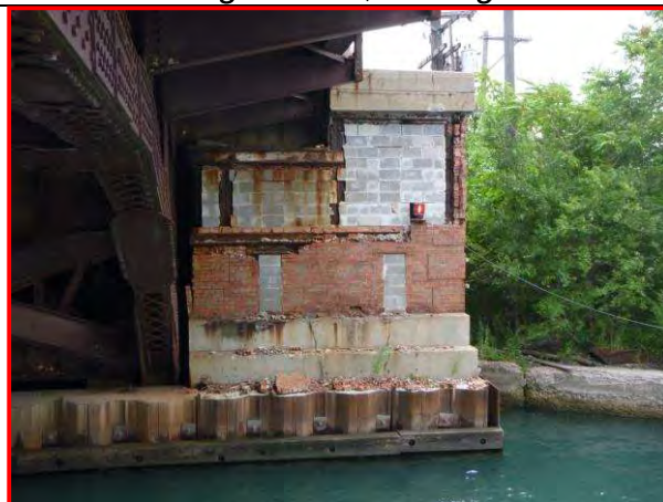
53. East bridge house, looking east
