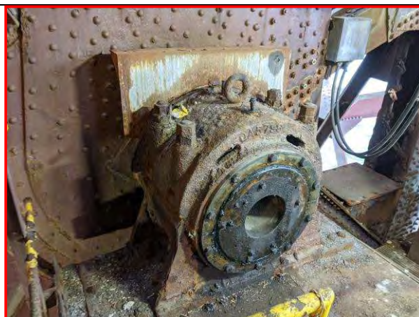
27. Southwest trunnion bearing, looking north
