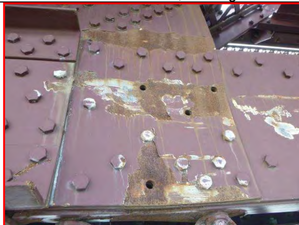
40. Bottom chord 2-4NW, looking south
