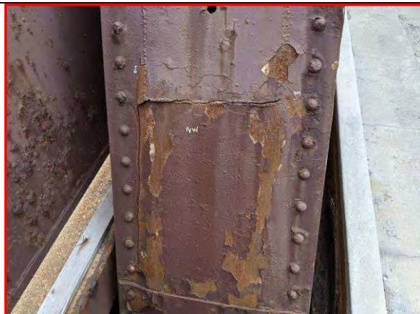
47. Northwest curved truss member, looking east
