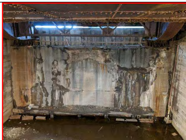
61. East face of west pit wall, looking east
