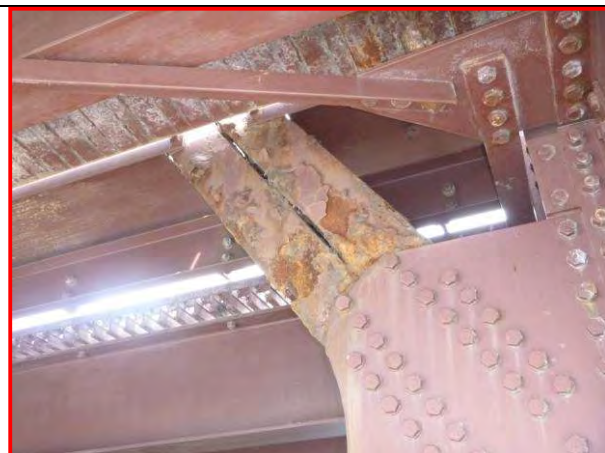
41. Diagonal 12-15SW, looking northwest
