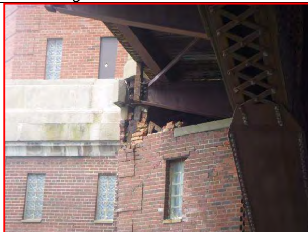
52. West bridge house, looking west
