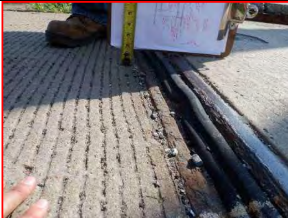
17. East Expansion Joint, looking south
