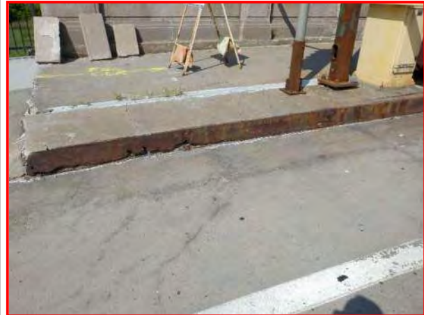
7. North curb plate in Span 4, looking north
