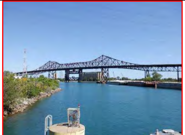
97. Upstream, looking north
