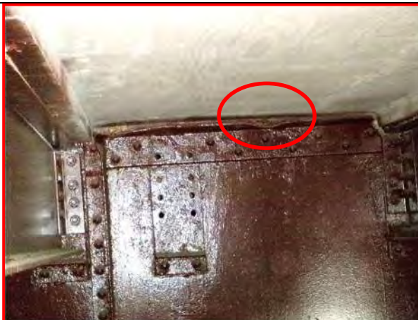
50. Floorbeam 21-21W, looking west
