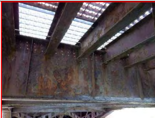
51. Floorbeam 8-8W, looking west
