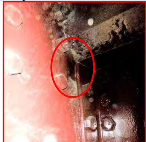
88. East Anchor Column Floorbeam, looking northwest
