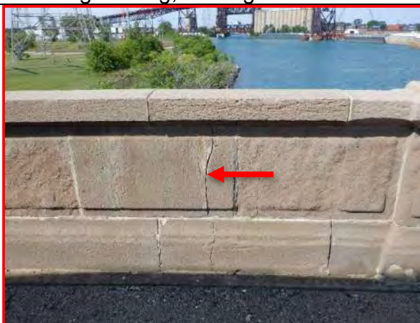
6. Stone parapets, looking north
