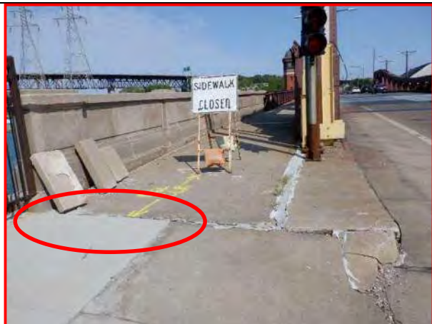
12. Northwest approach sidewalk, looking east
