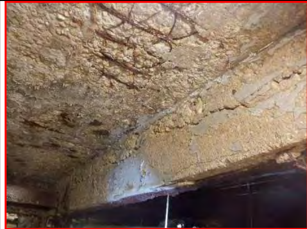
44. Span 4 sidewalk stringers, looking northwest
