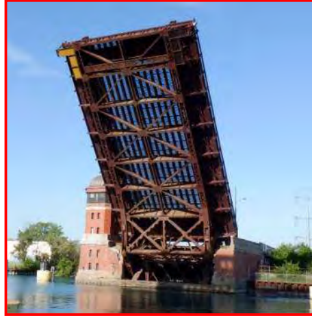
38. Overall underside of the movable span, looking southwest
