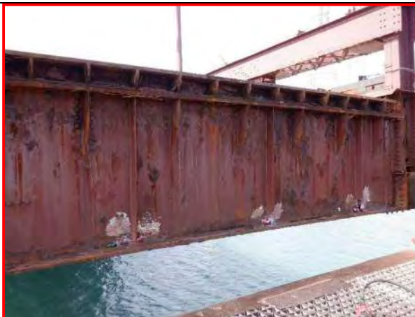
55. FB 0-0W, looking northwest
