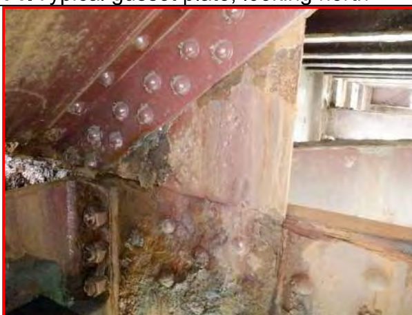
72. Northwest inside face gusset plate at Panel Point 0, looking southeast
