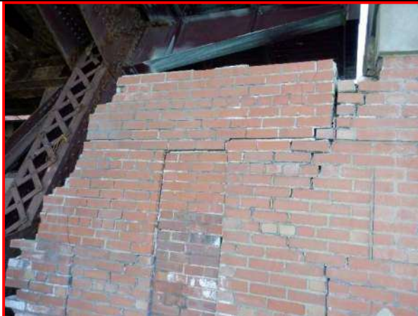
77. North enclosure wall at West River Pier, looking west
