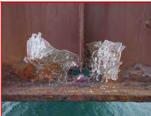
54. FB 0-0E crack, looking east
