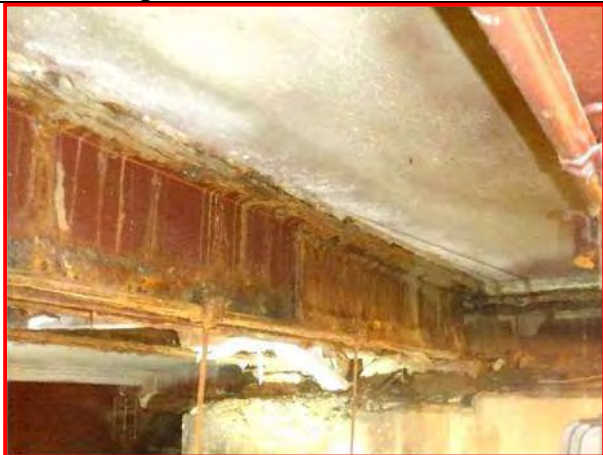
43. Span 5 north sidewalk stringer, looking southwest
