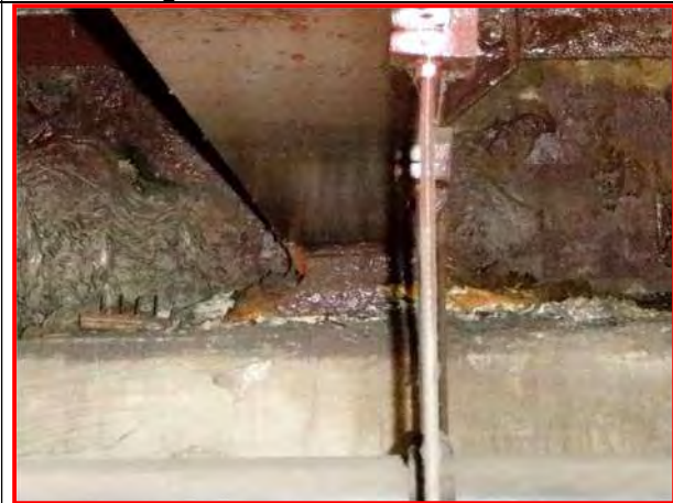
39. Typical West Abutment Bearing, looking west
