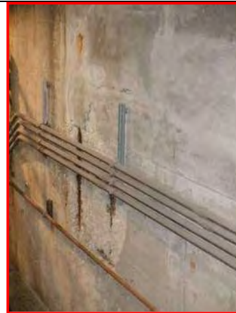
82. West Abutment elevation, looking southwest
