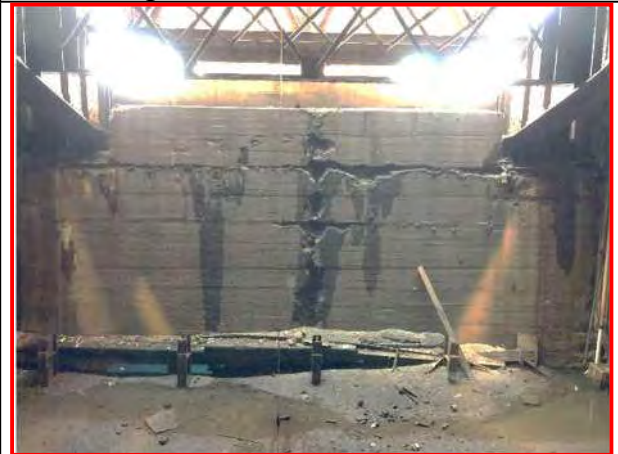
86. East River Pier counterweight pit face, looking west
