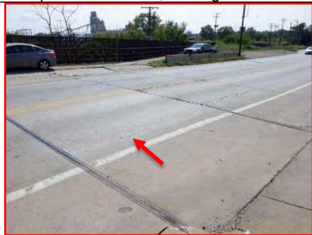
30. West Approach, looking southwest
