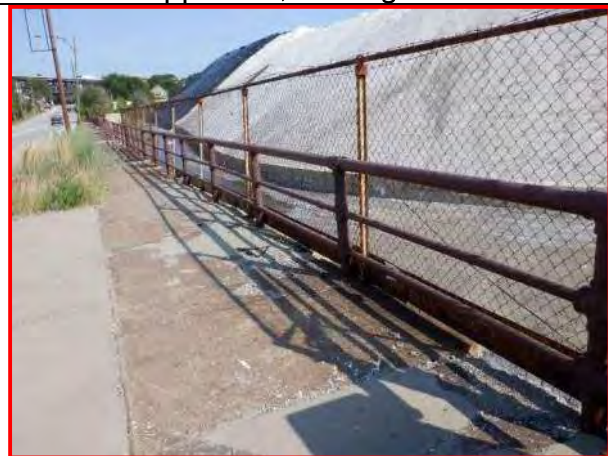
31. Southeast Approach sidewalk, looking east
