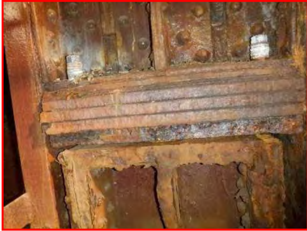
42. Typical secondary live load bearing, looking east
