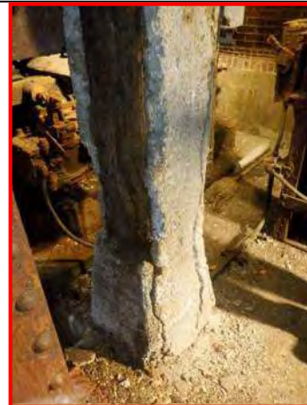
90. Sidewalk column near the Southwest Anchor Column, looking southeast
