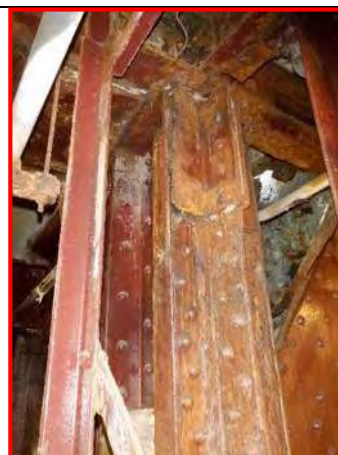
96. Sidewalk column paint system, looking north
