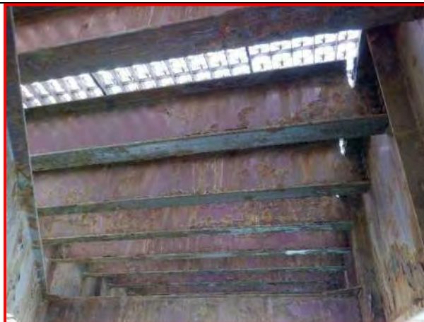
95. Superstructure paint system, looking north
