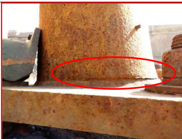
15. South light standard in Span 5, looking south
