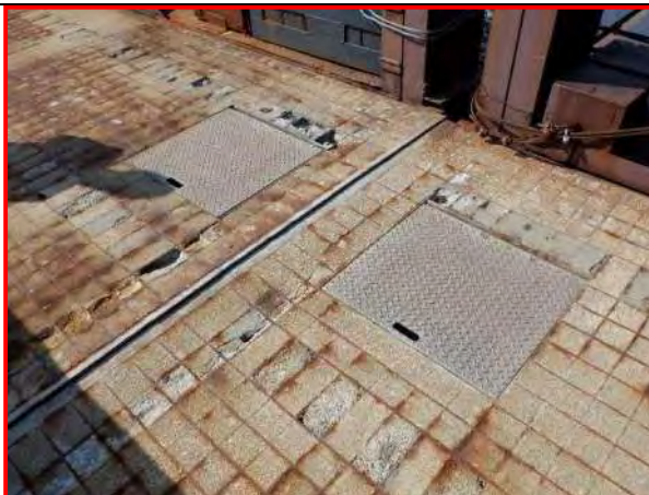
21. South sidewalk at the center break, looking northwest
