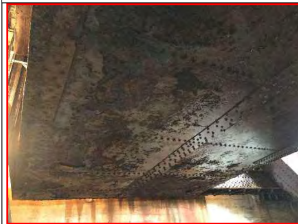
76. East counterweight box, looking south
