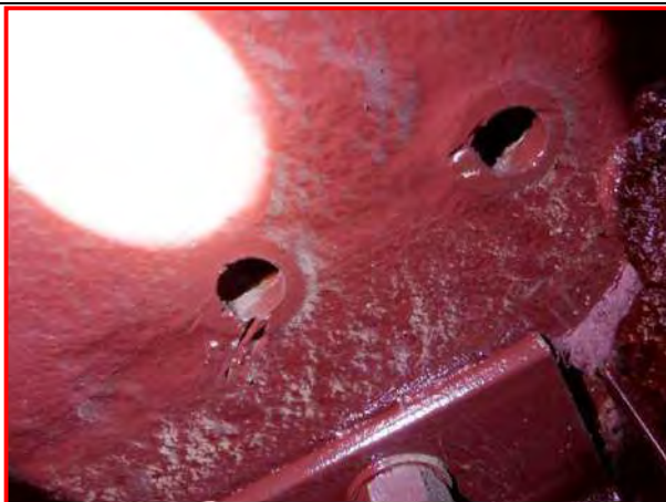
87. West Anchor Column Floorbeam, looking east
