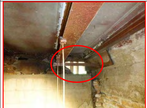
83. West Abutment backwall, looking west
