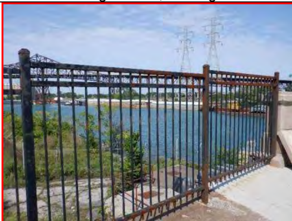
33. Northwest approach fence, looking northeast
