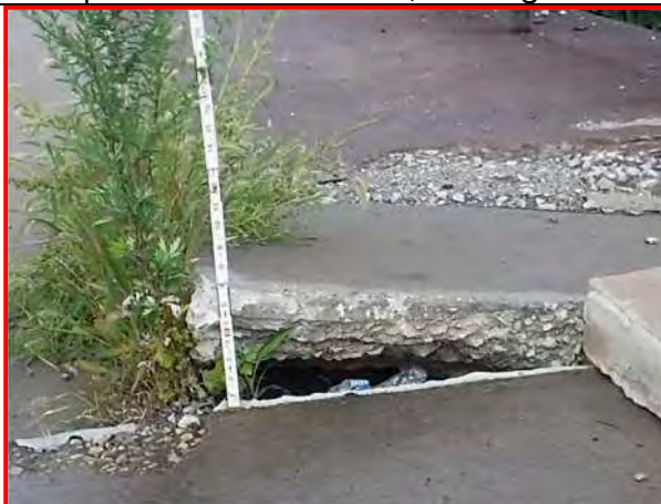
11. Northwest approach sidewalk during the 2019 inspection, looking west
