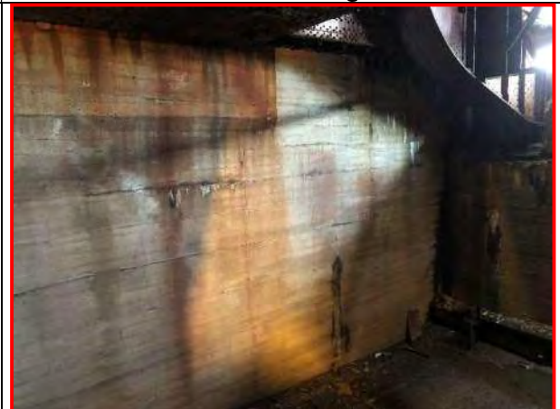
91. East Counterweight Pit South Wall, looking southwest
