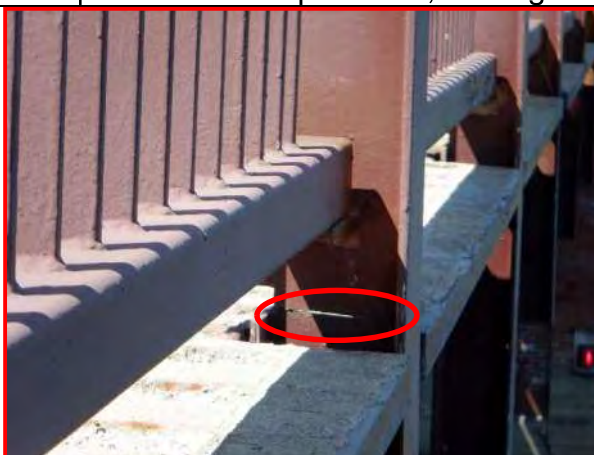
5. Bridge railing, looking west
