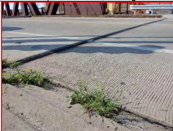
18. East Expansion Joint, looking northwest
