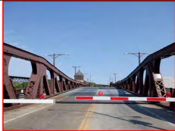
1. Overall top of deck, looking east
