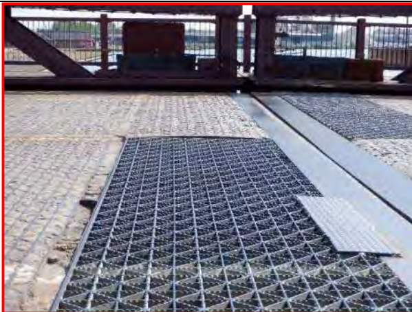
2. East leaf near the center break in Span 3, looking south
