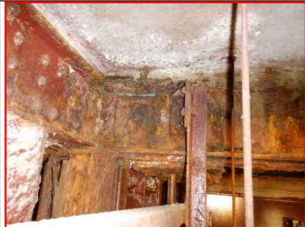
45. Connection between sidewalk stringer and floorbeam in Span 5, looking south
