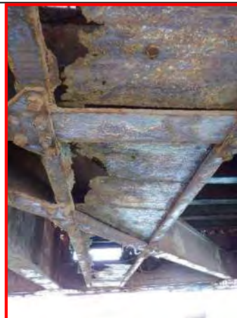
81. Catwalk steel plate near Floorbeam 2-2W, looking north and up
