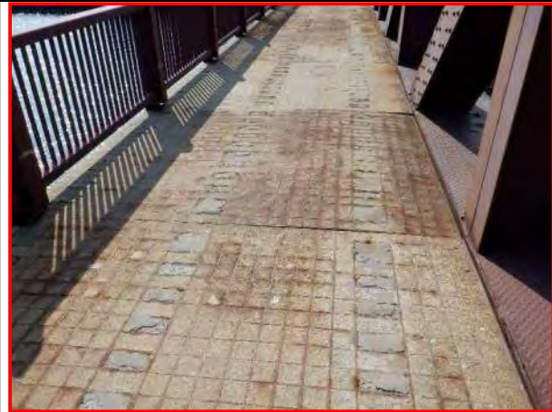
8. South sidewalk in Span 3, looking west
