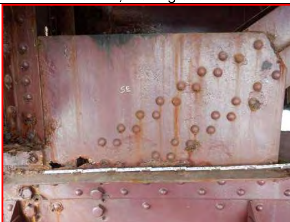
74. Southeast outside face gusset plate at Panel Point 0, looking north
