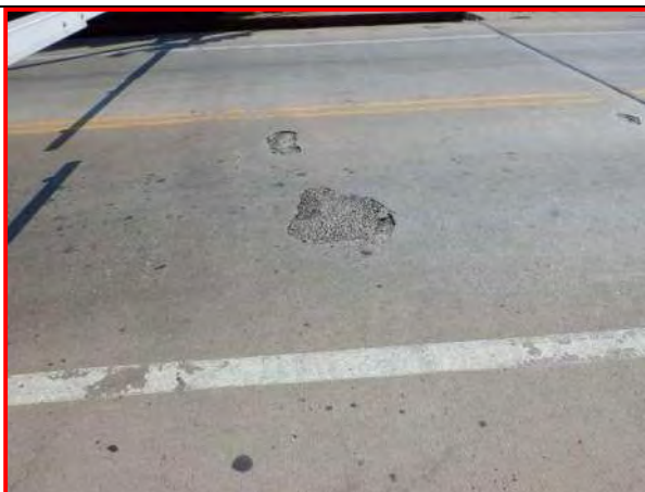
4. Spans 4 and 5 top of deck, looking south
