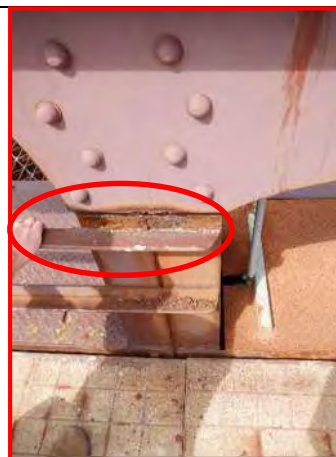
70. Weld on vertical member of southwest truss, looking north
