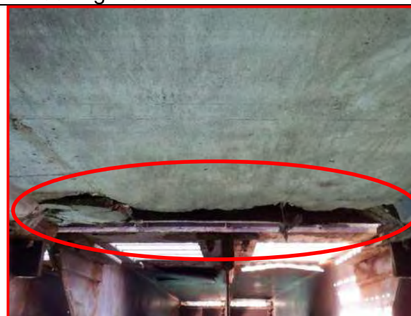
28. Span 2 deck soffit, looking west
