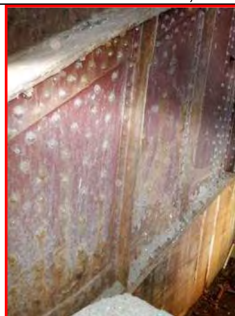
49. Southwest Trunnion Girder end, looking southwest
