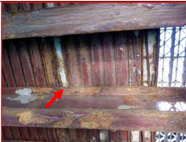
25. Metal pans in Span 3, looking up
