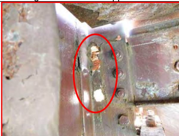
46. Span 3 curb stringer, looking west
