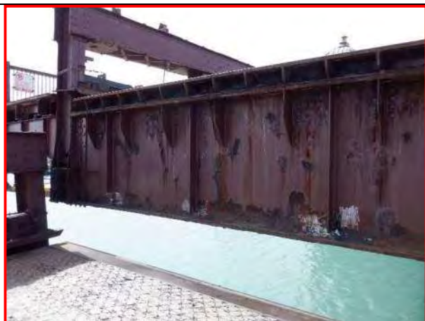
56. FB 0-0W, looking southwest
