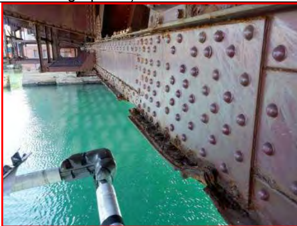
65. Northwest Truss Member 2-4, looking east
