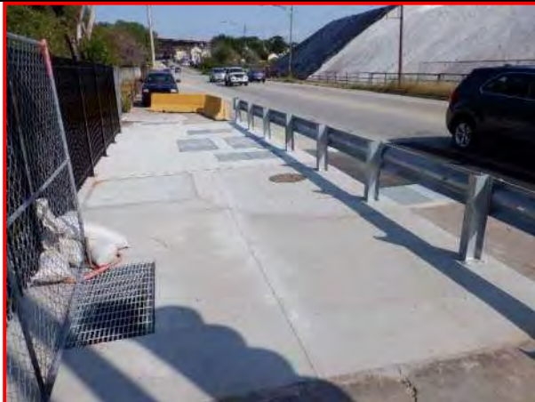
32. Northeast guardrail, looking east
