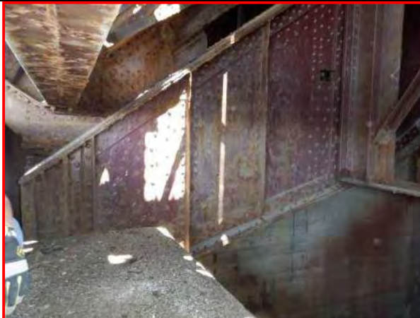
48. Northeast Trunnion Girder, looking north
