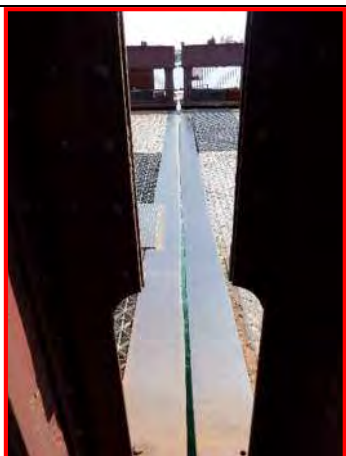
19. Center break, looking south
