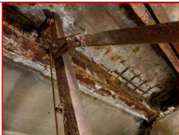
27. Span 1 sidewalk soffit, looking up
