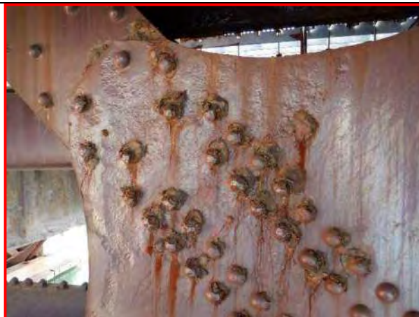
71. Typical gusset plate, looking north
