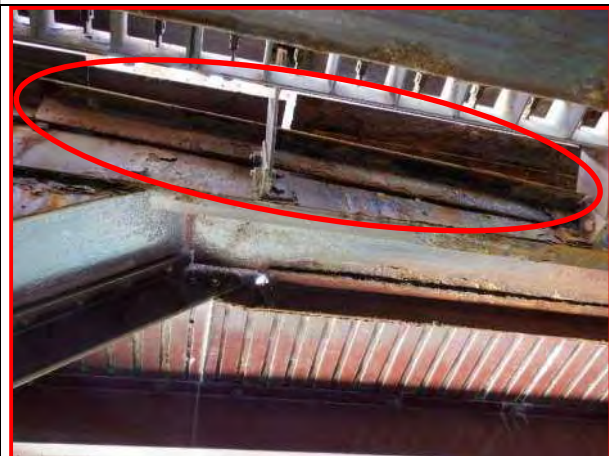
47. Top flange angle at the curb stringer, looking up
