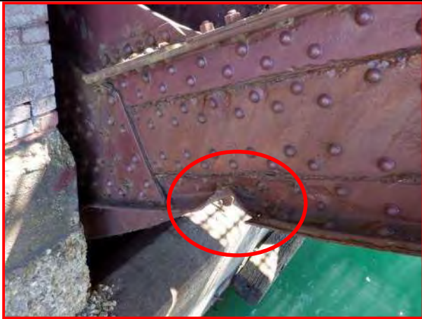
62. Northeast Truss Member 12-14, looking south
