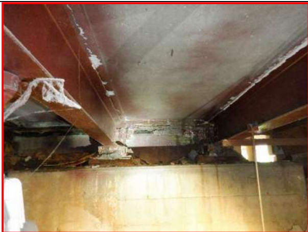
61. Span 5 sidewalk diaphragm, looking west
