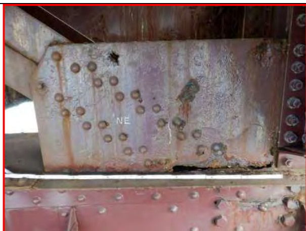
73. Northeast outside face gusset plate at Panel Point 0, looking south
