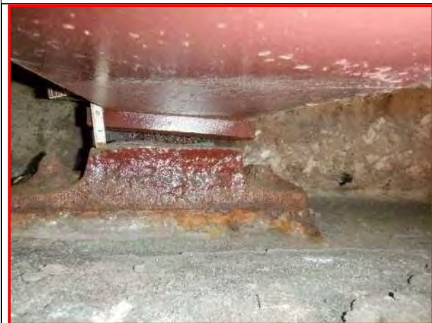
40. Span 1 Stringer S6 bearing, looking east
