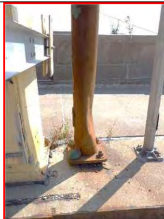
14. South light standard in Span 5, looking south
