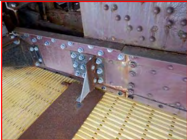
64. Southwest Truss Member 0-2, looking north
