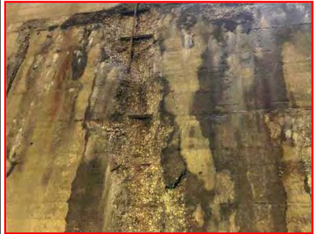
85. West River Pier counterweight pit face, looking east
