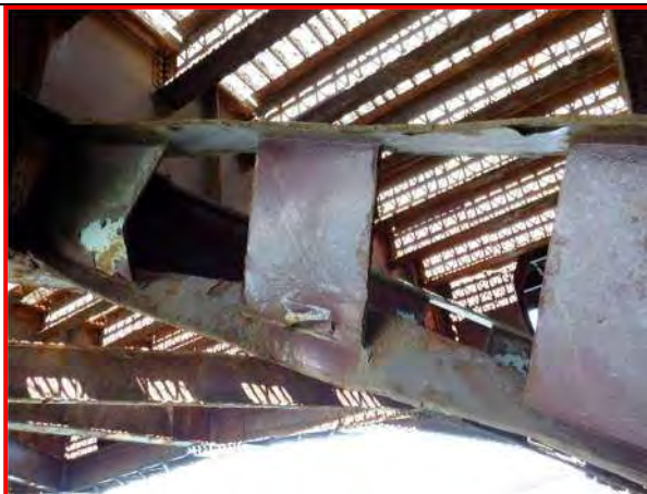
58. Span 3 Panel 1 lateral bracing, looking north
