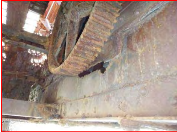
63. Northwest Truss Member 0-2, looking southeast
