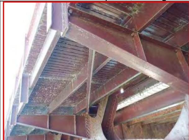
9. North sidewalk soffit in Span 3, looking southeast
