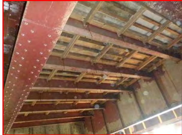
29. Span 4 deck soffit, looking northeast
